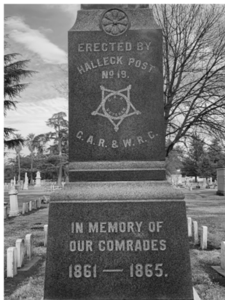
Figure 9 - Front view (south-facing) of the two dark gray granite blocks. Note the polished and unpolished surfaces, the engraved 5-pointed star symbol, and the embossed “flower” at the top of the upper block.
