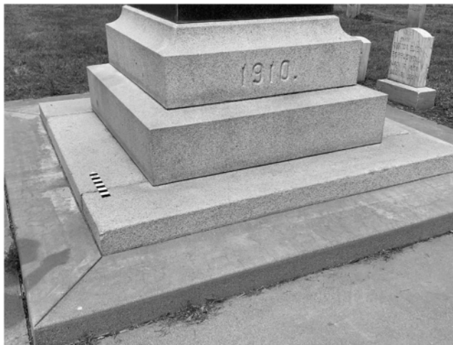
Figure 7 - View of the three light gray granite slabs forming the lower section of the pedestal along with the concrete border (step) which abuts the lowest light gray granite slab. The one-foot-long north arrow rests on the bottom slab. Note the fitted parts of the bottom light gray slab. The inscription "1910." was engraved on the front (south) face of the top slab.
